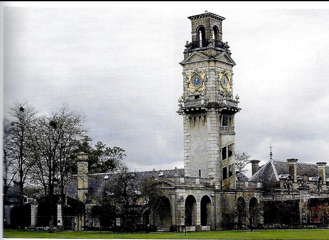
Fig 3.9 The Italianate water tower, Cliveden. Water was piped to tanks in the tower from a farm on the far side of the River Thames by steam- powered pumps.
