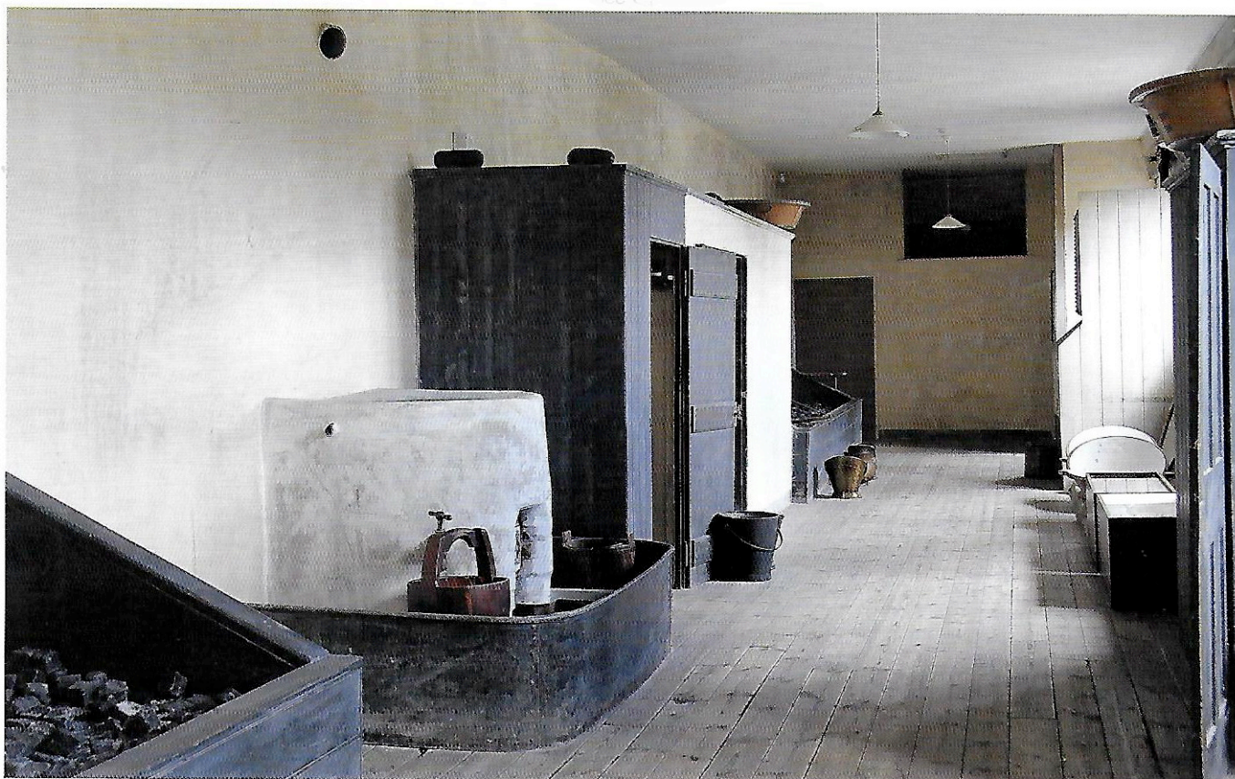
Fig 3.12 The Coal Gallery on the second floor at Audley End, with a 19th-century copper for hot water supplies and bins for storing coal, which was raised from the gardens below by a hoist.
